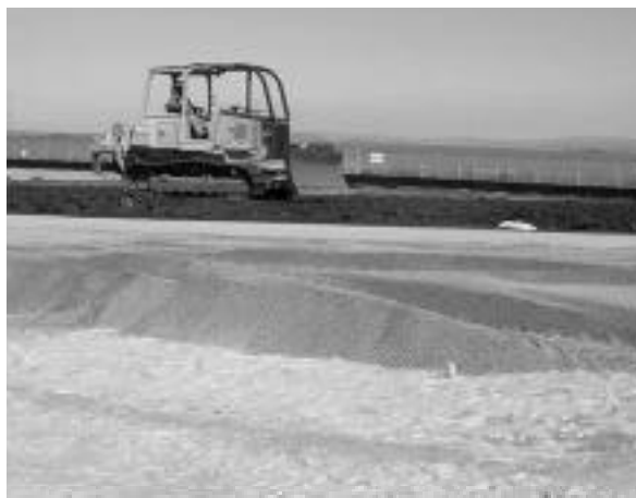
Loader installs soil layer of biotic barrier.
