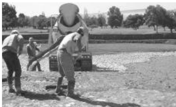
Workers place slurry along grids.
